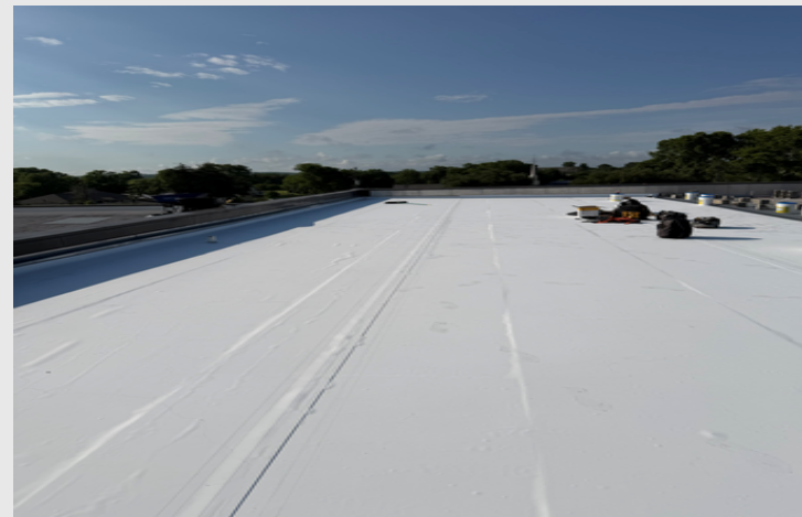
Reroof over ES locker rooms
