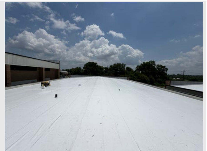
Reroof over Current Elementary School
