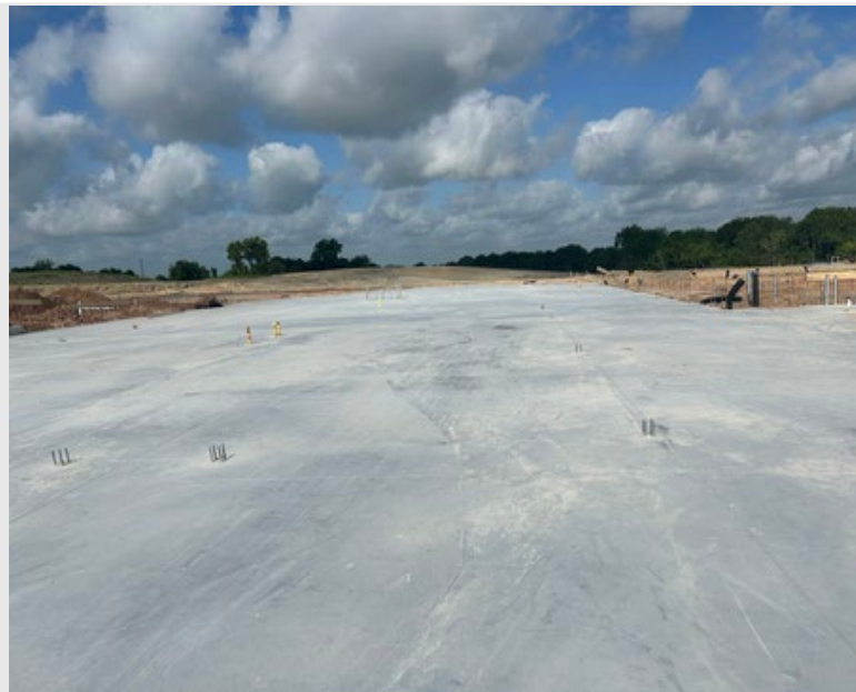
Area C Foundation (Cafeteria)
