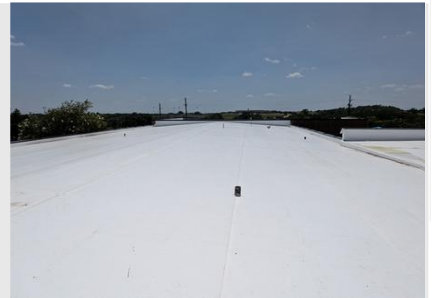
Completed re-roof current ES
