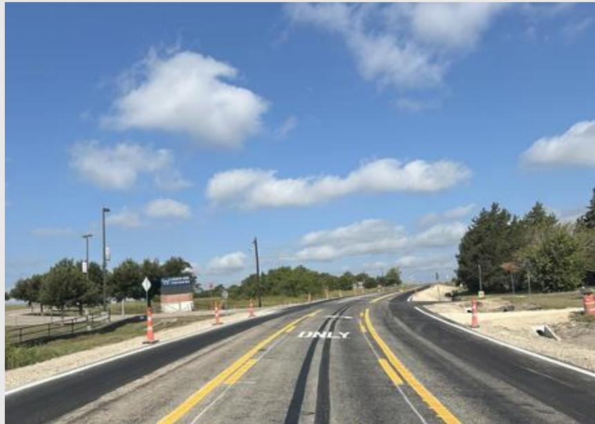
FM-149 Road Widening
